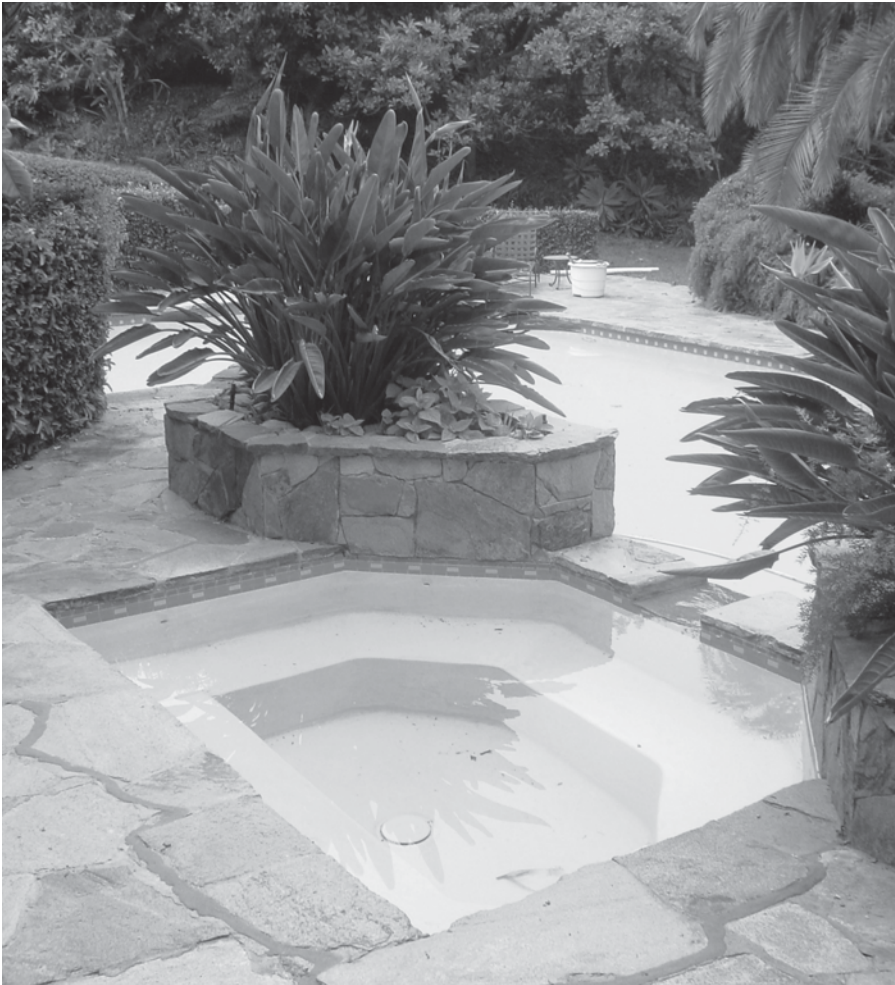
FIGURE 1-23B The finished pool and spa.
