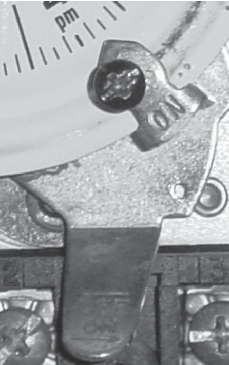
FIGURE 7-2 (A) Typical electromechanical time clock; (B) on/off tripper; (C) visual inspection port on time clock; (D) typical twist timer.
