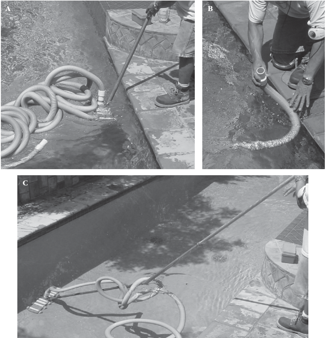
FIGURE 9-8 (A) Preparing the vacuum; (B) preparing the hose; and (C) vacuuming the pool.
