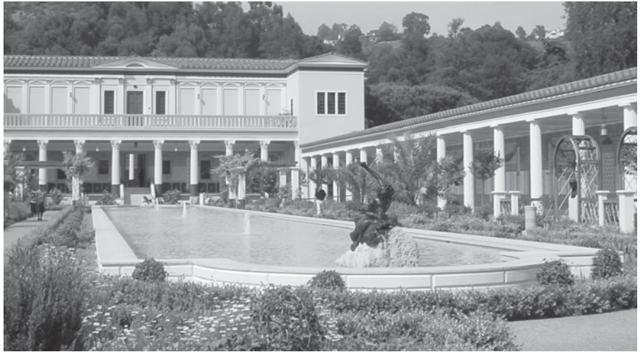
FIGURE 1-8 In-ground concrete pool.
