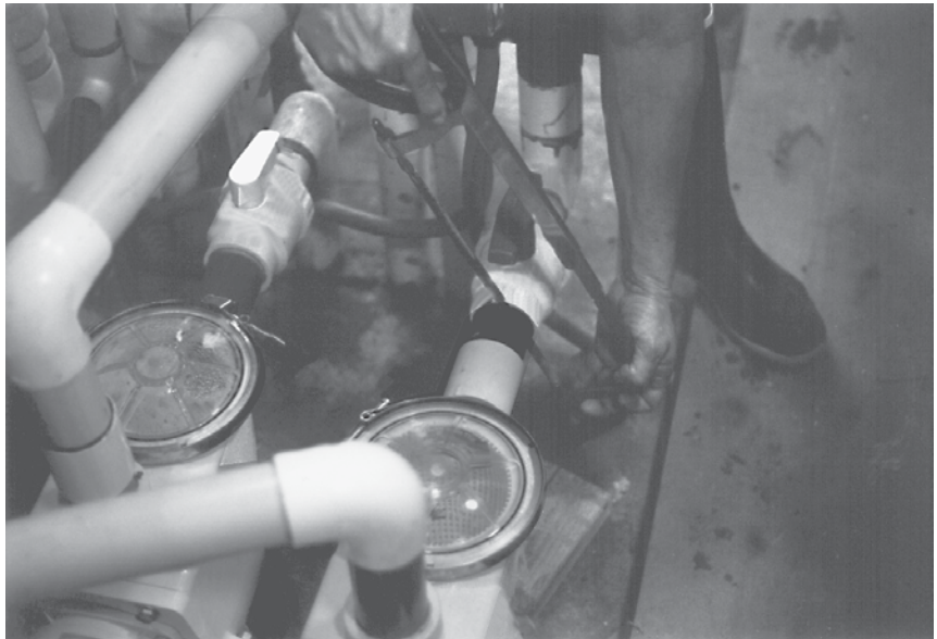
FIGURE 4-13 Pump and motor removal.
