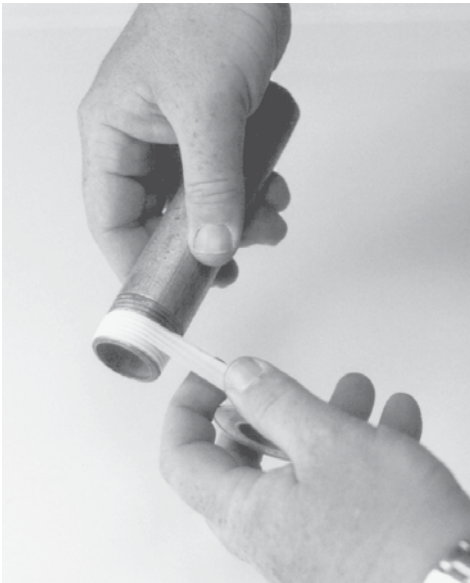
FIGURE 2-8 Correct application of Teflon tape.
