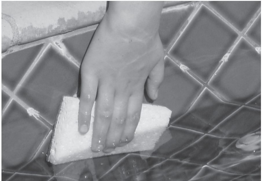
FIGURE 9-7 Scrubbing the tiles.
