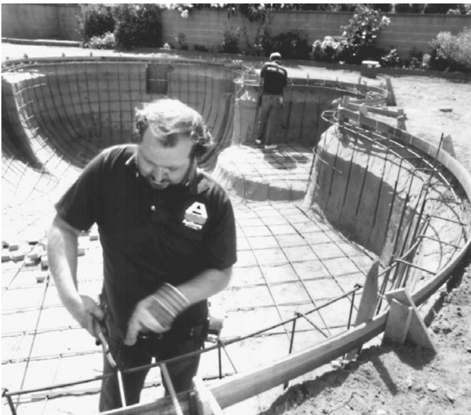
FIGURE 1-17 Typical phases of pool construction. Anthony & Sylvan Pools, Doylestown, Pa.
