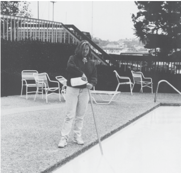
FIGURE 9-11 Adding glycol to main drain.
