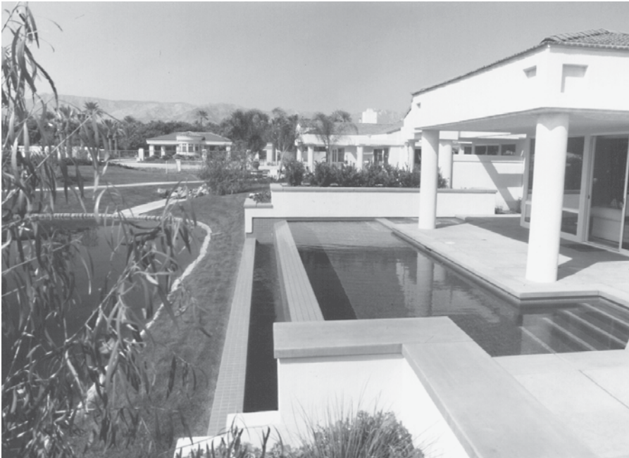
FIGURE 11-4 Vanishing edge pool and catchment basin. California Pools & Spas, West Covina, Calif.
