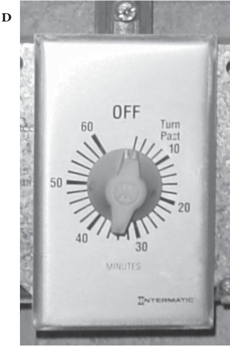
FIGURE 7-2 (A) Typical electromechanical time clock; (B) on/off tripper; (C) visual inspection port on time clock; (D) typical twist timer.
