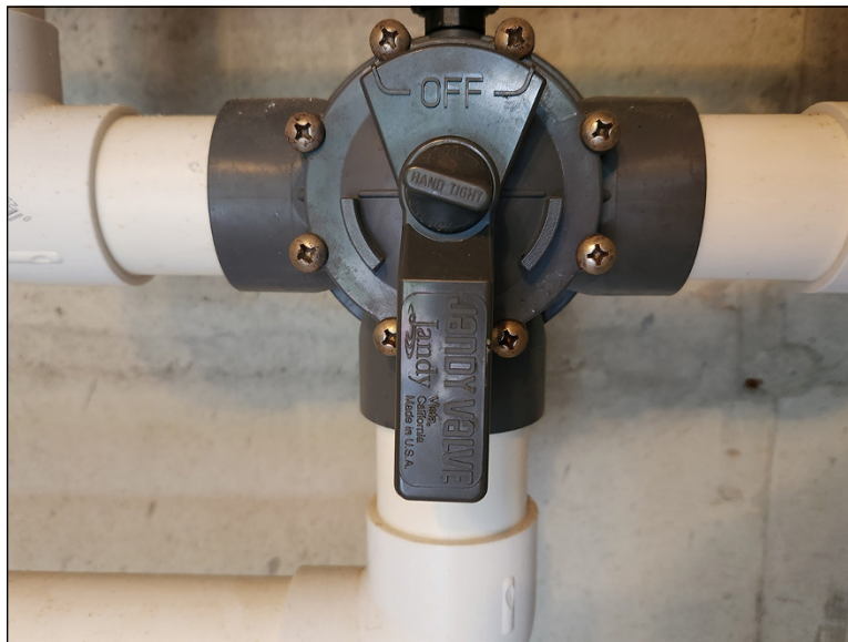
FIGURE 3-2: A 3-way valve that controls a skimmer (left) and a main drain (right) that goes to the pump (bottom).
