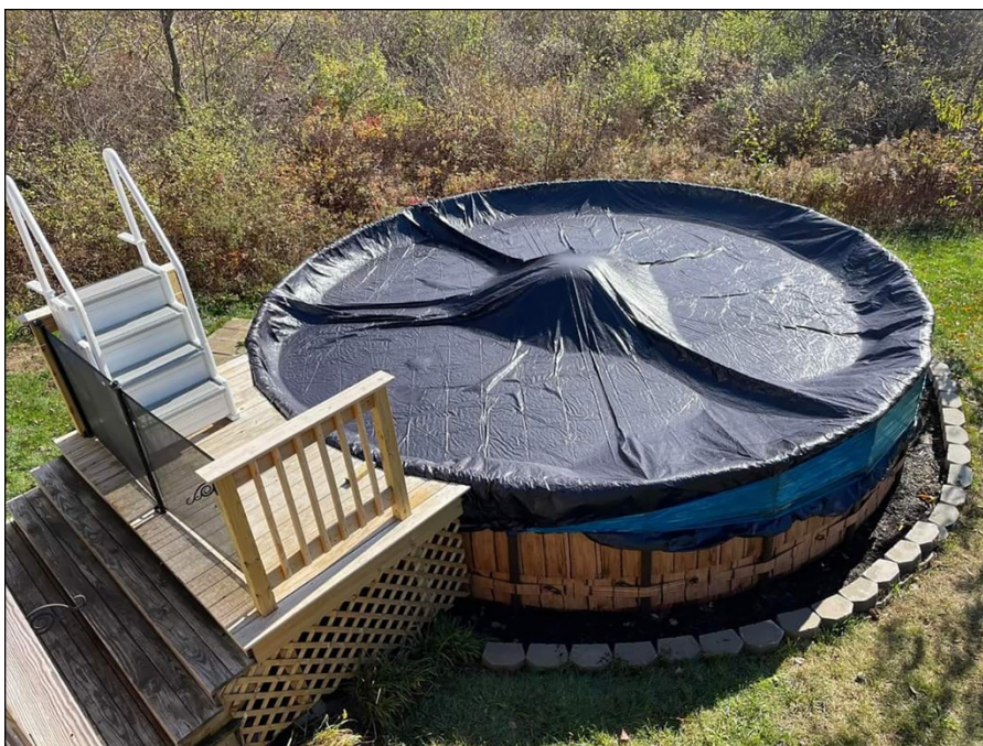
FIGURE 8-3: A cover properly installed on a pool that doesn't get a lot of snow — it fits but with very little slack.
