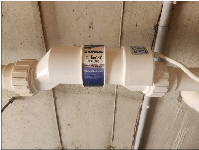
FIGURE 3-4: A Hayward T-Cell 15, a very common salt cell.
