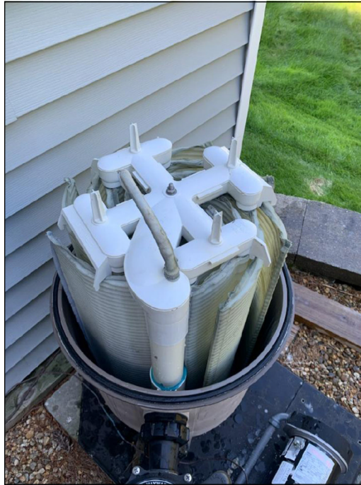
FIGURE 3-11: The inside of a grid-style DE filter.
