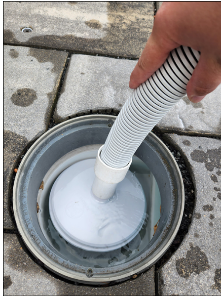
FIGURE 7-5: Place a vacuum plate attached to the vacuum hose into the skimmer.
