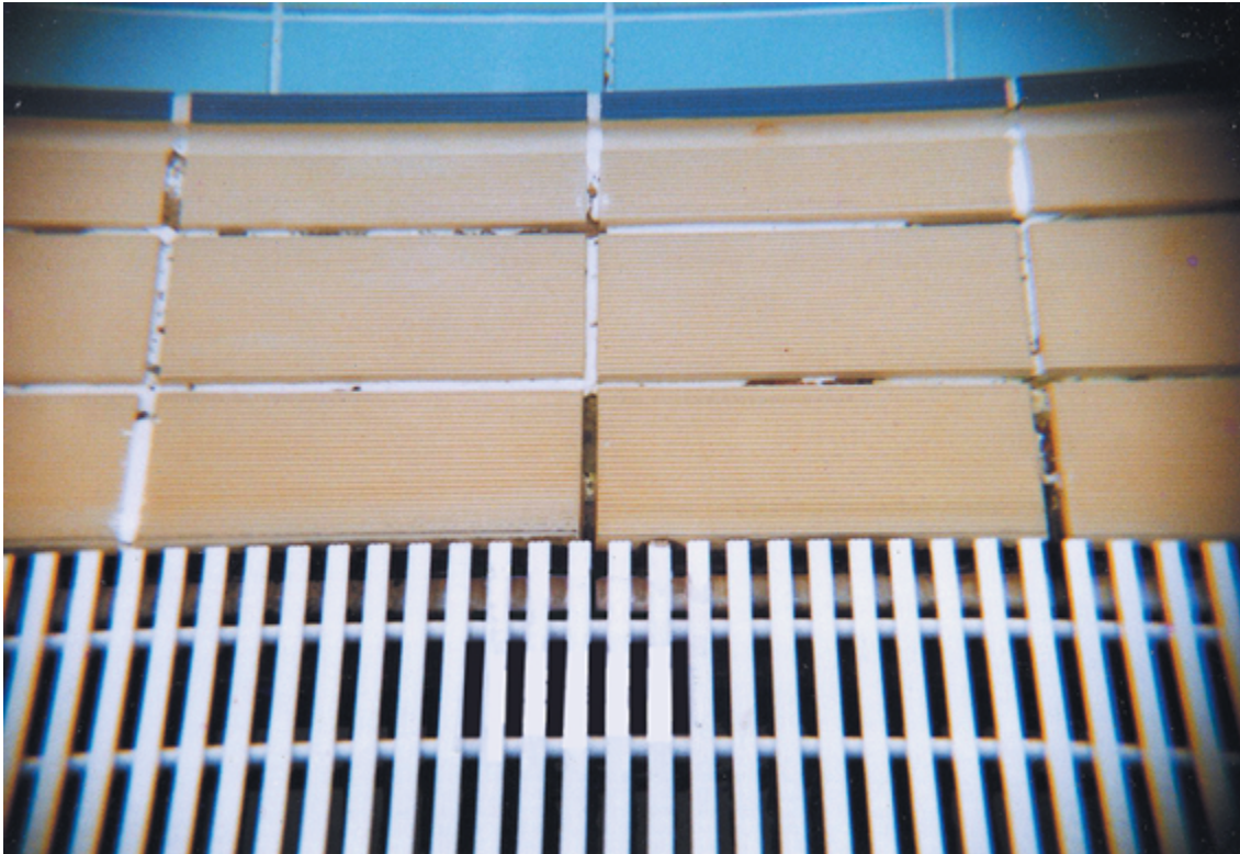
Photograph of Cement Screed of Tiles Etched at the Overflow Edges of a Pool Figure 9-2
